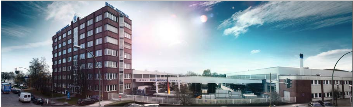
JORDAHL's registered office and administrative headquarters on the premises of its affiliate PUK
