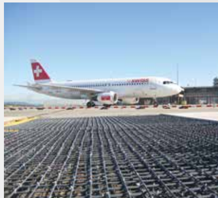
Airport Zurich <Switzerland >
