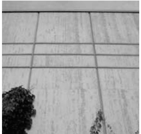
CHAMFERED COVE, DEEP IN CONCRETE
