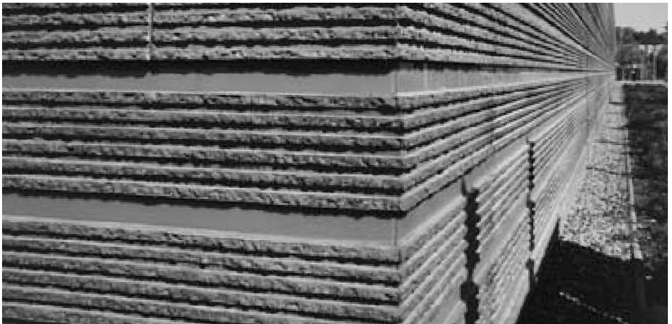
COVE WITH CHAMFER, MIDDLE IN CONCRETE
