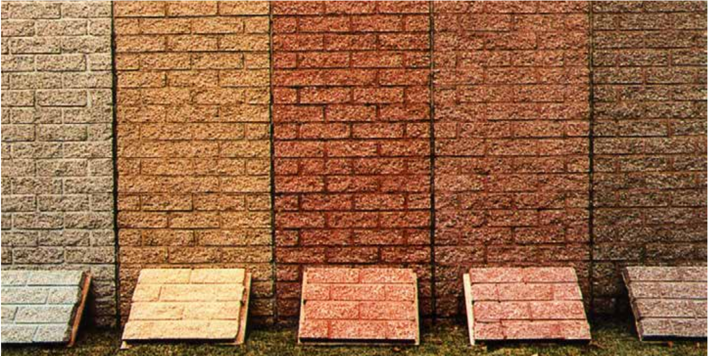
Fig. 18: Concrete walling blocks after 25 years of outdoor weathering
