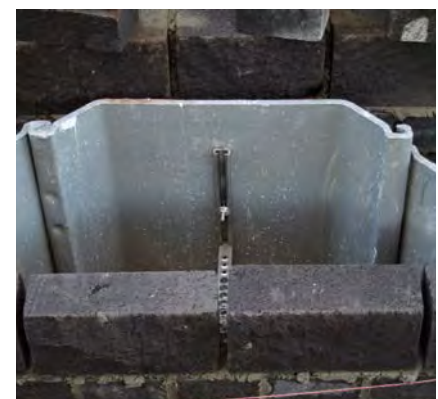
Connection of facing masonry to bulkhead wall
