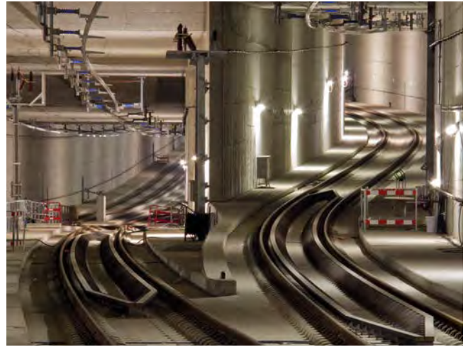
City Tunnel, Leipzig, Germany
